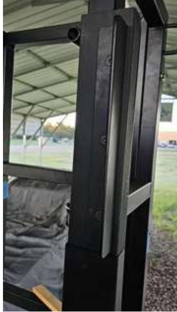
Window Rake Station
